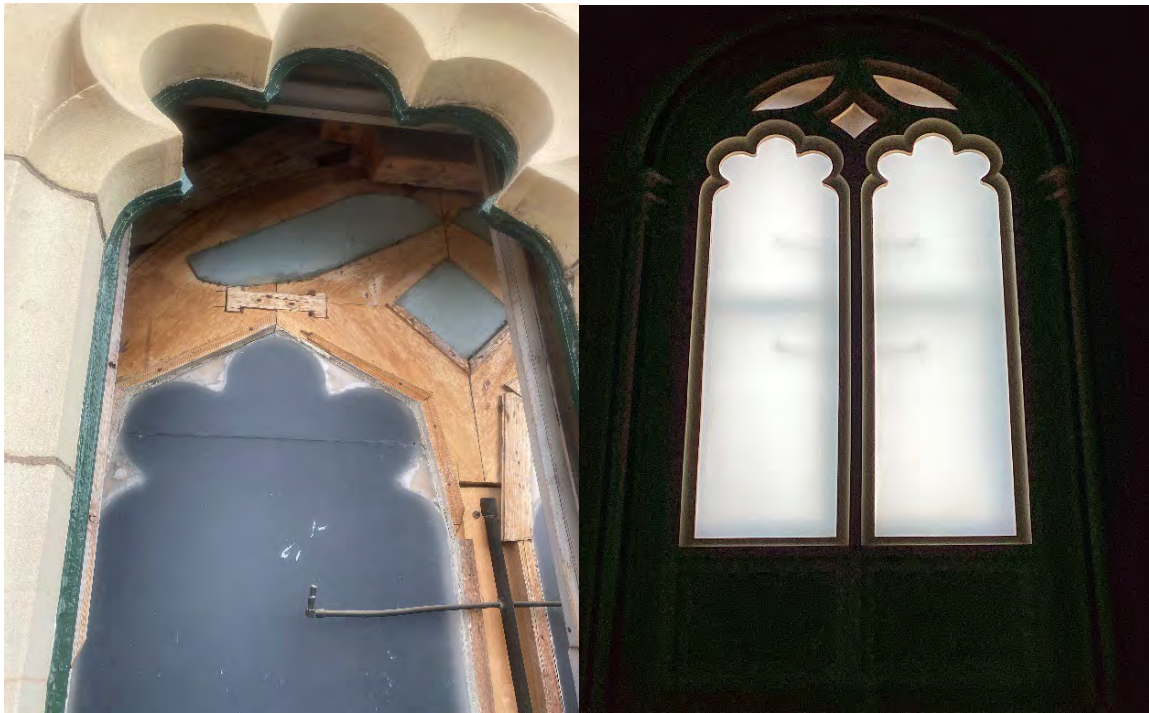
Original glass from within the cavity and the new laminated glass installed as viewed from inside the Ball Room
