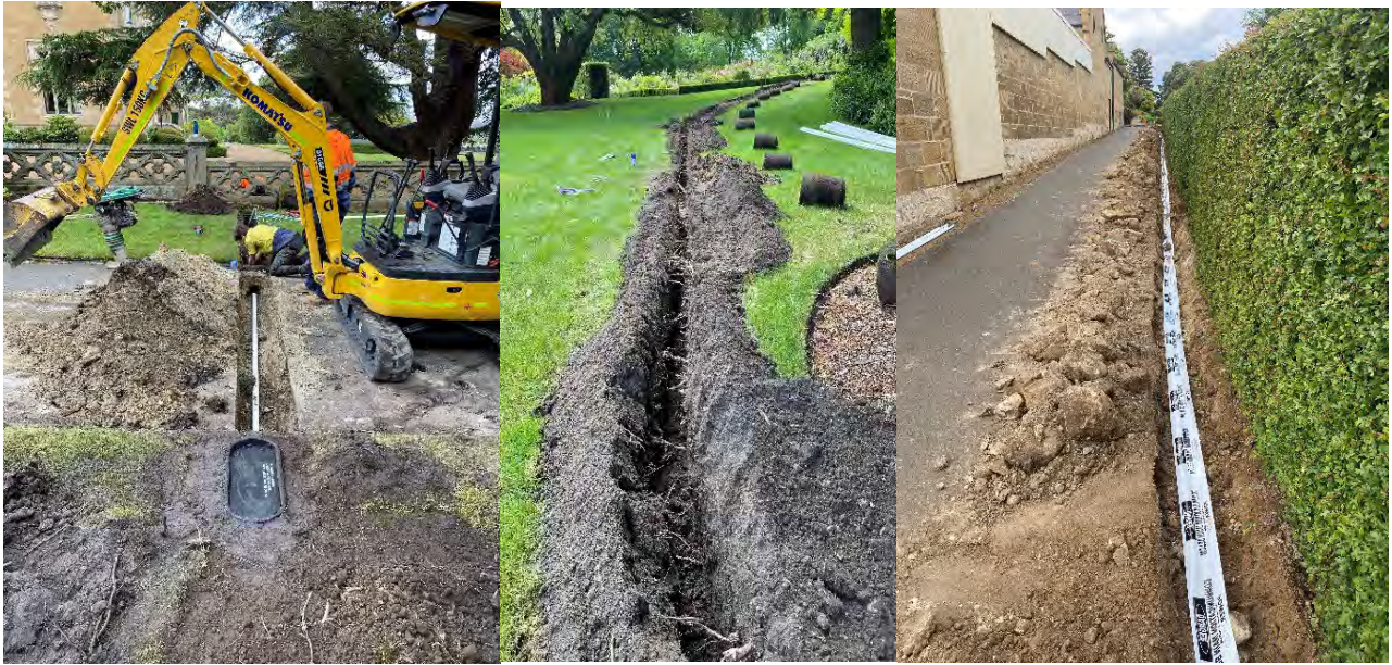
Excavation work for security upgrade
