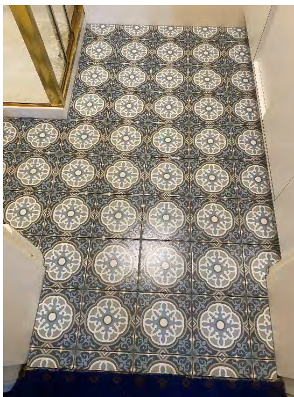
New tiles to Franklin bathroom floor
