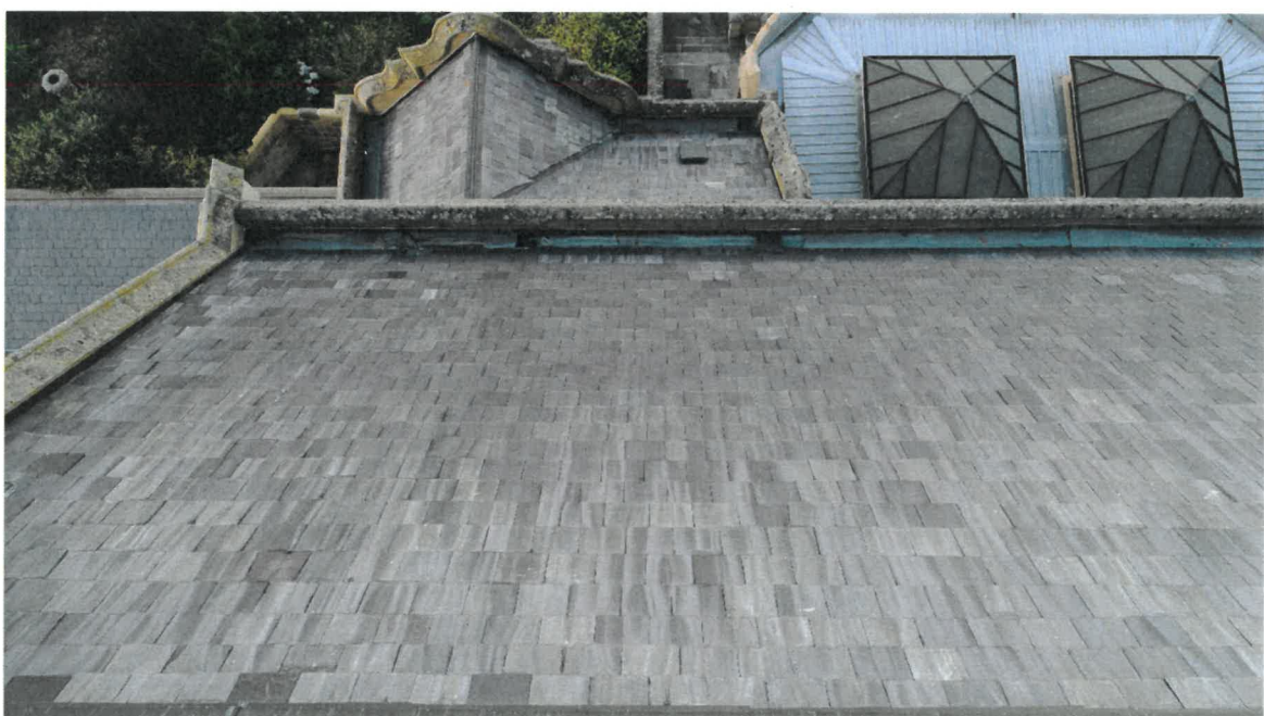
Drone technology enables effective monitoring of gutters and Welsh slate tiles, March 2018
