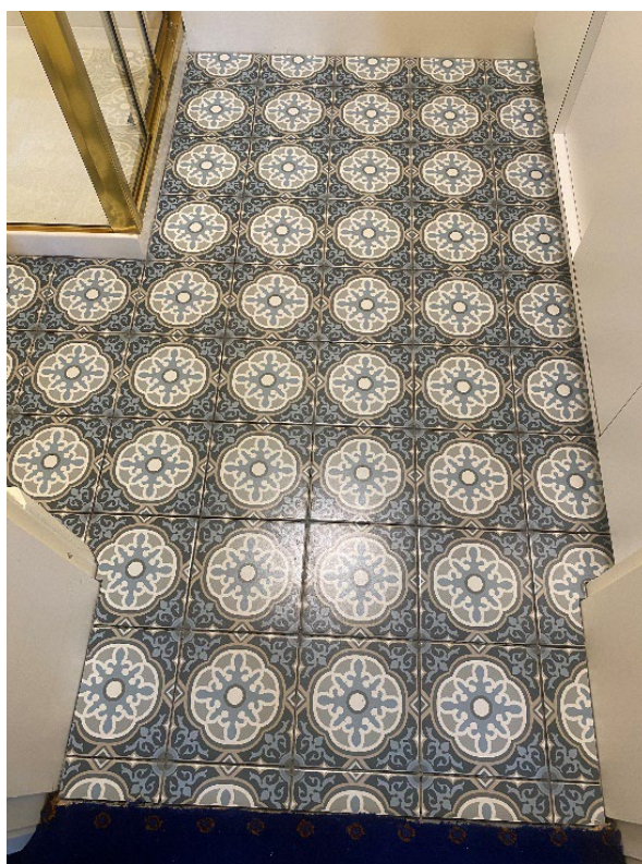
New tiles to Franklin bathroom floor
