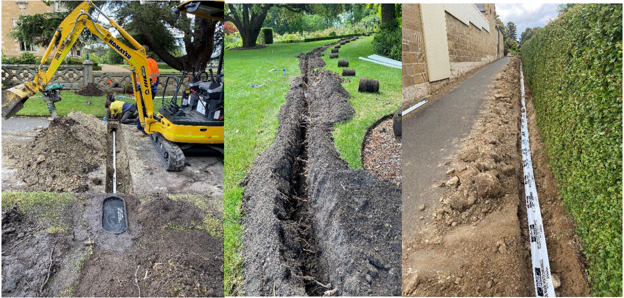
Excavation work for security upgrade
